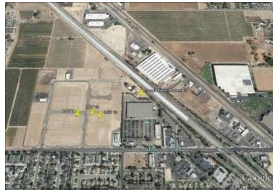
Aerial view of Kingsburg Business Park.
